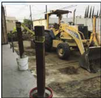
Preparing the ground for paving.
