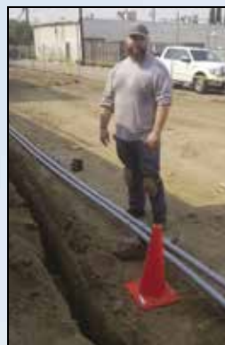
Trench for burying the cables.
