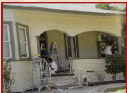
GARDEN house before renovations
